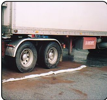
Peat Booms protecting a stormwater drain
